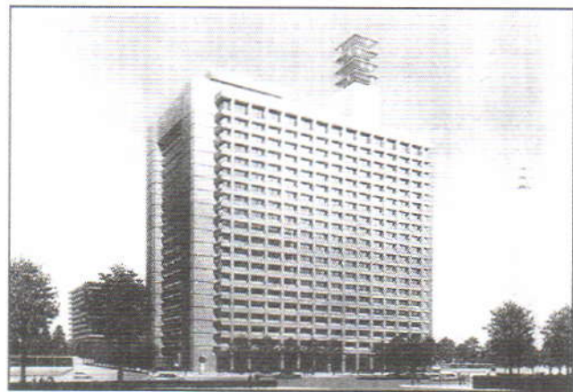
Fig. 13 Central government building (with HD + VD) (Courtesy of Kume Sekki Co. Ltd.)
