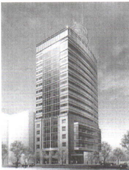
Fig. 20 DoCoMo Nagano (with VD) (Courtesy of NTT Power and Building Facilities Inc.)
