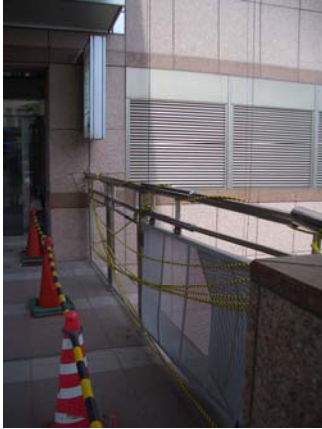
Photograph 3.7 Expansion joint of the bridge.
