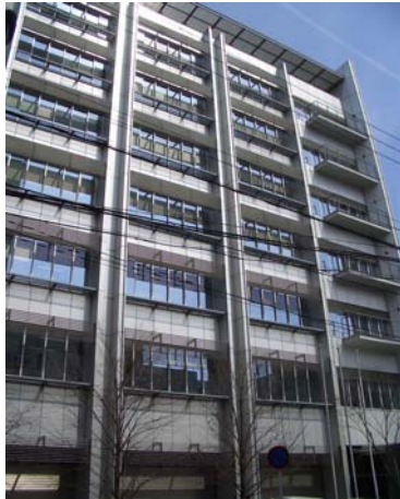
Photograph 3.1 Appearance of Building F.
