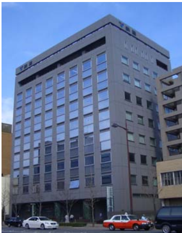
Photograph 3.4 Appearance of Building G.
