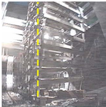
Photo 9. Loss the stability of frame just before collapse
