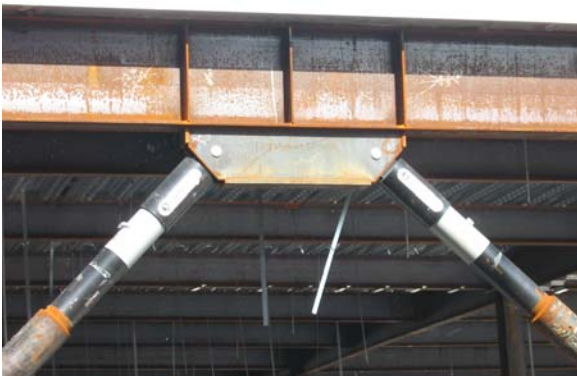
Figure 1. steel moment frame with dampers
