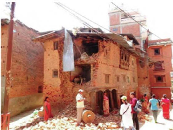
Fig. 1. Unreinforced masonry building damaged in the Gorkha earthquake in 2015 [3].
