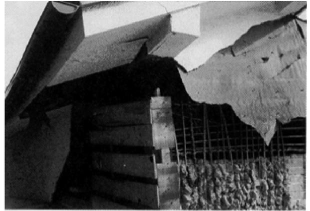
Fig. 8. Connection failure of a wooden house in the Great Hanshin Earthquake in 1995 [8].
