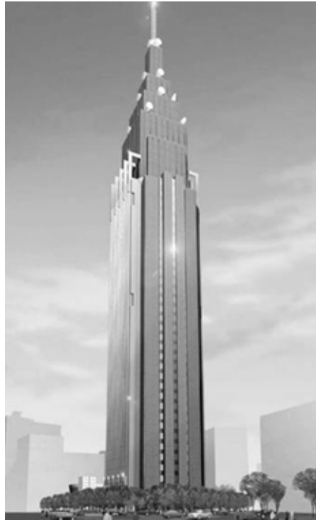
Fig. 10 DoCoMo Tokyo Building (with viscous damper) (courtesy of NTT facilities).
