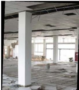
Figure 19. Damaged suspended ceiling
