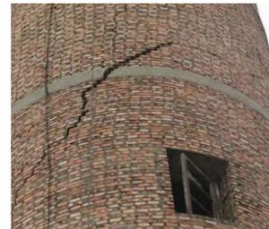
Figure 29. Shear crack in URM water tower
