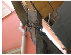
Figure 10. Column flexural failure
