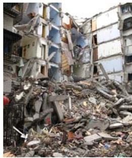
Figure 20. Collapsed corner of the building
