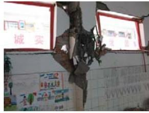
Figure 9. Captive column failure
