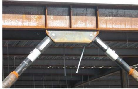
**Fig.1:** Viscous dampers used for design of a new building in California
